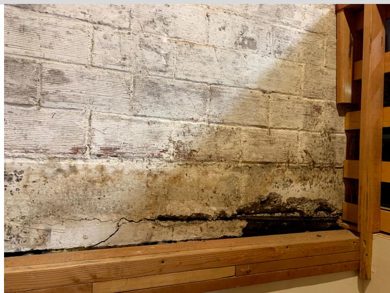
The conditions of our current City Hall & Police Station building are well below what would be expected from a facility housing public safety, emergency management or other critical municipal operations. Some of the structural walls are made from hollow block. This building material is known to have minimal abilities to withstand the forces generated by earthquakes. The building shows ongoing settlement issues.
