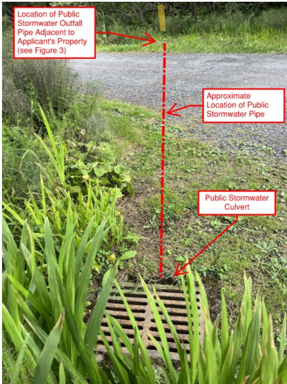
Figure 2: Public Stormwater Catch Basin (west side of Forest Lawn Road, looking east)
