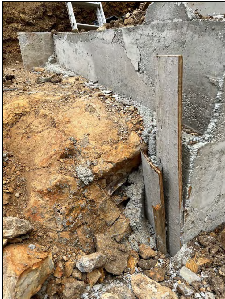
Photo 3: Bedrock exposed during construction. View looking northwest towards Ash Street.
