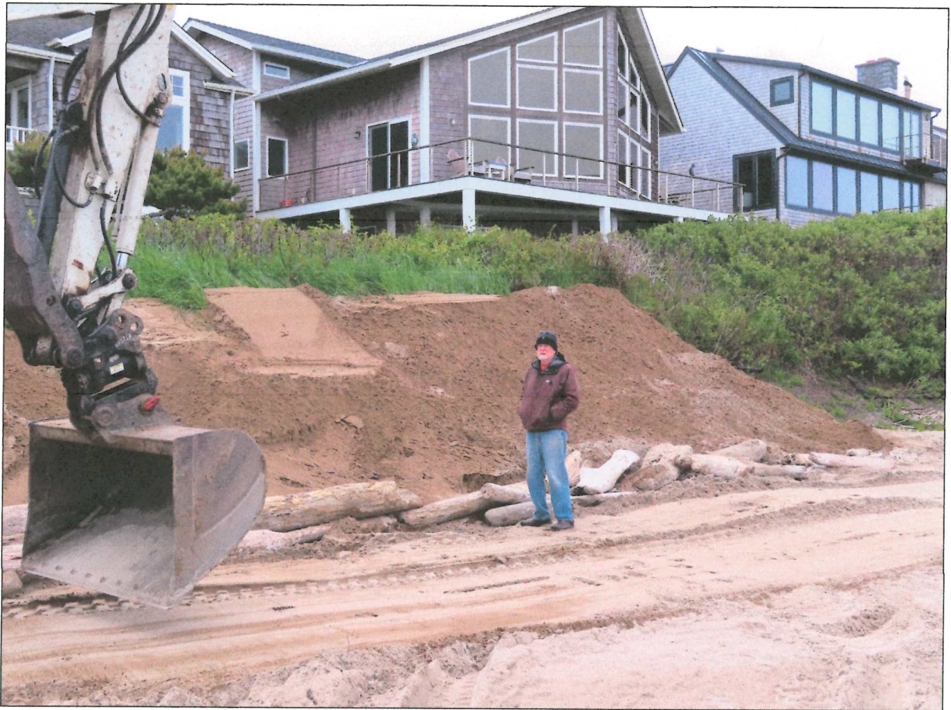
Figure 4: Freshly placed sand over round rock basalt cobbles to repair gap in face of the frontage berm from the storm surge of January 3, 2022. Photo taken May 27, 2020. Mike Morgan provides scale.
