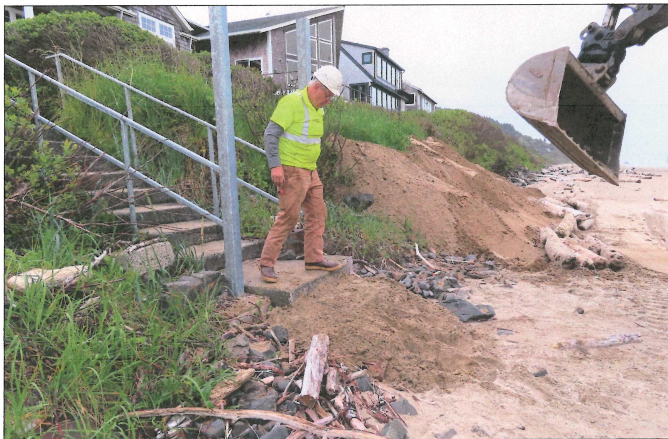
Figure 3 : Placing sand at the toe of the neighborhood steps and over obscured round rock, looking south. Mike McEwan provides scale.
