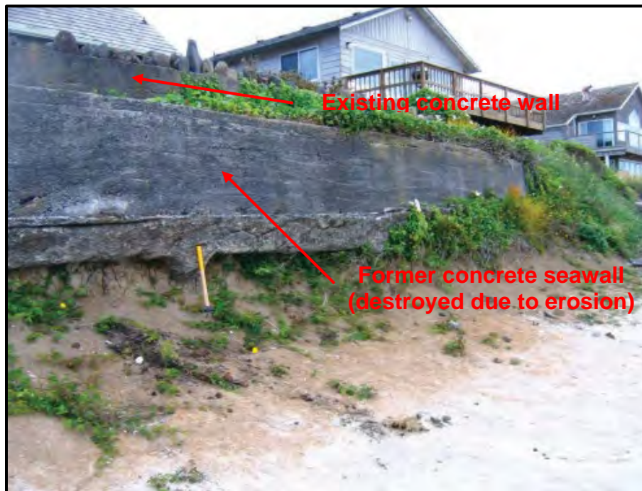
Photo 2: Undated photo of site beachfront and former seawall, presented in Witter et al (2009) as an “example of a seawall in Cannon Beach that has been undermined by wave erosion”.
