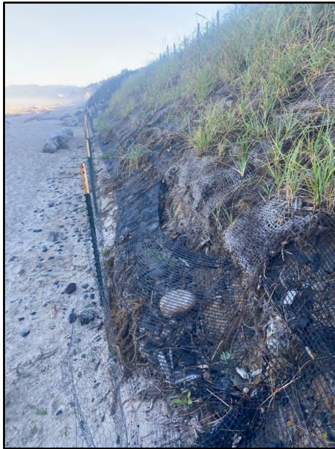
Photo 5. Looking north at the sand burrito-type SPS, installed in 2021 on the western edge of TL 2200. Note the substantial observed vegetation denuding and erosion that has occurred in the course of one winter season.
