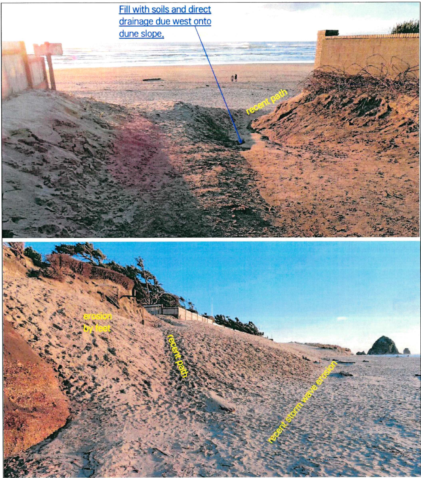
Figure 6: Top: View to west along right of way of West First Avenue. Pedestrian traffic and water flow have caused erosion to shift to the north side of the route and sculpt a gully that veers to the north after passing the fence. This gully needs to be filled and a new route sculpted to keep water in the middle of the road. Bottom: View to south, showing a recent path by pedestrians, the foot traffic pushing sand down the slope toward the beach. Note the footprints in the open sand above the trail, erosion by feet. The upper beach has been anomalously eroded, probably removing at least 20 ft of foredune, exposing terrace gravels on lower left. Compare with dune sands in Figure 5. Signage or fencing will be needed to direct foot traffic around this sensitive eroded area. Photos dated February 22, 2022.
