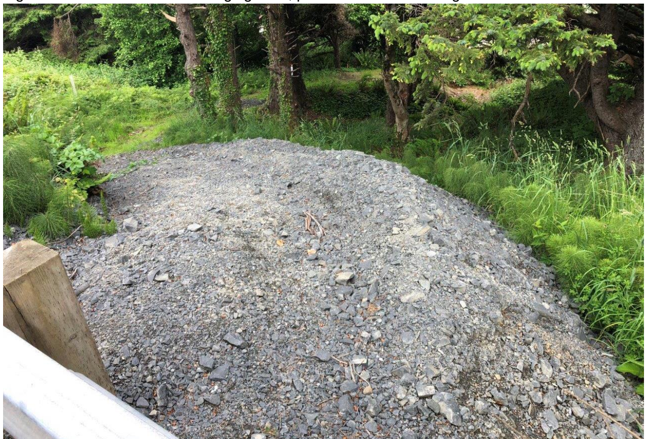
Photo 1 – Photo of well-graded aggregate temporary access ramp in place, provided by PLI.
