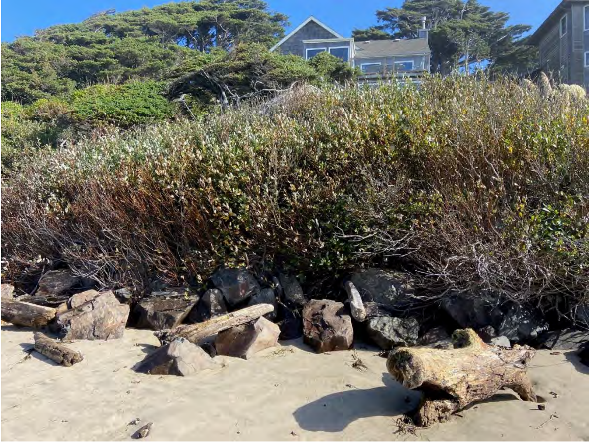
Site Photo, October 18, 2023
